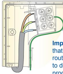
**Important!** Make sure that the inlet earth wire is routed as shown. Failure to do so may cause product malfunction.
