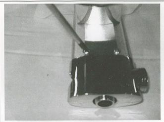
Remove the two screws, you will then be able to remove the bottom section
